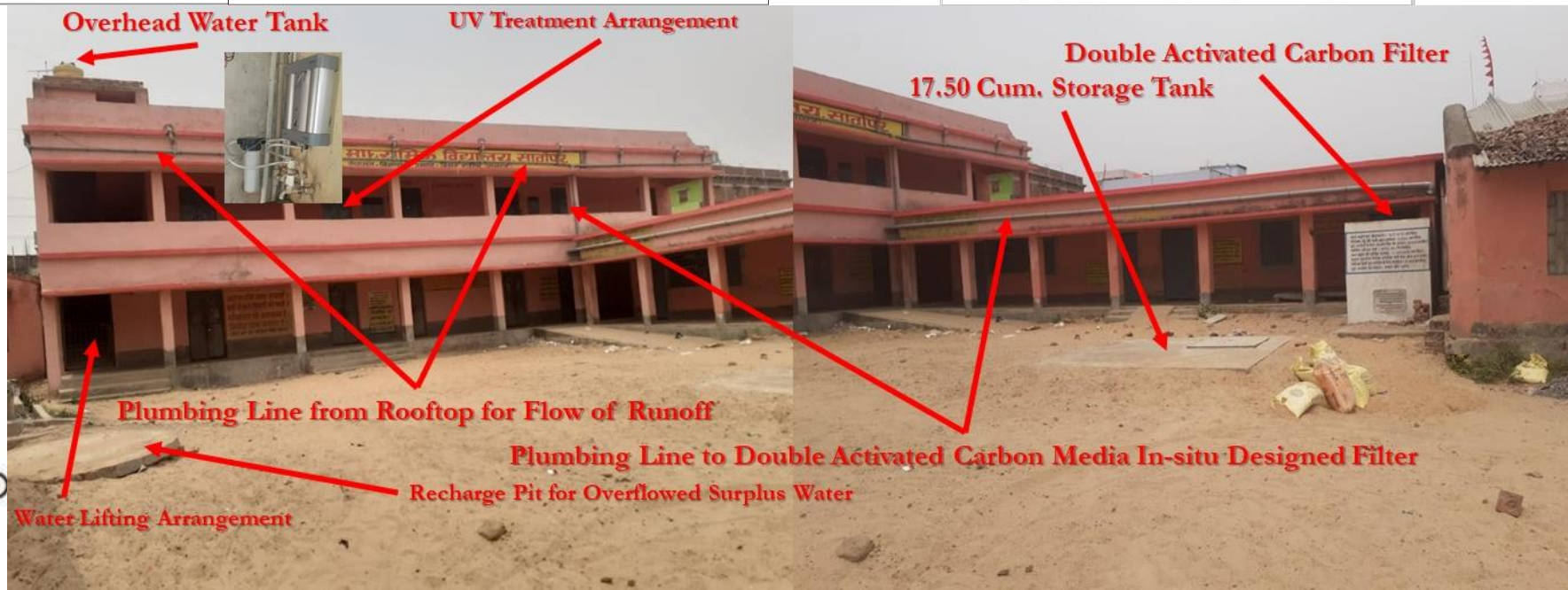
Plan of Recharge Pit for Rooftop Rainwater Harvesting System
